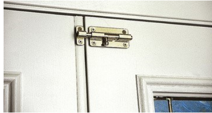
FIGURE 53-6 A slide lock is at the top of the door. The person is not likely to look for a lock here.
